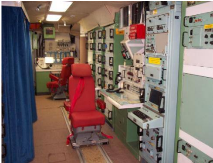
Launch Control Center Delta-01
