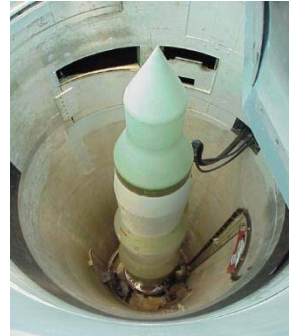
Launch Facility Delta-09
