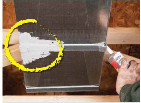
Seal ducts at joints to prevent heated or cooled air from leaking out or unconditioned air from leaking into the ducts.
