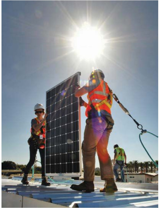
Solar panels can be installed on ground- or roof-mounted racks, and some products can integrate solar cells with the roof of your home.
