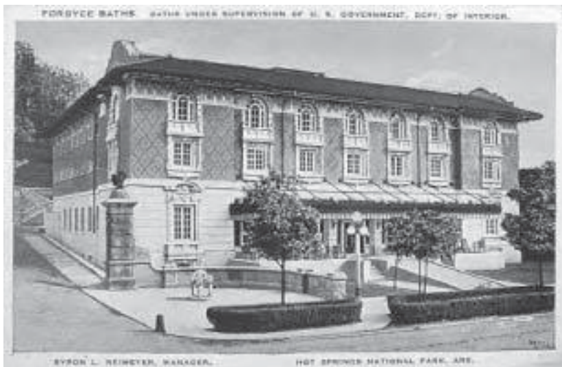
The Fordyce Bathhouse was the finest on Bathhouse Row when it was built in 1915.
