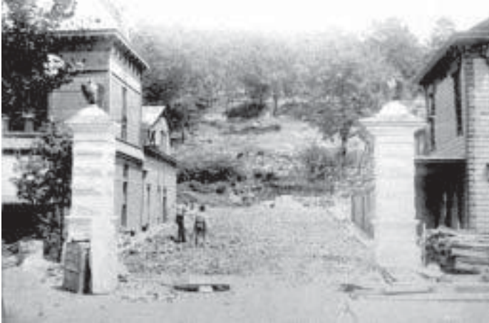
Grand Entrance —construction, 1893
